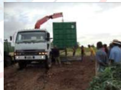
placing the two containers onto the foundations
