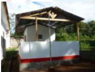
Newly built laundry & toilet facility
