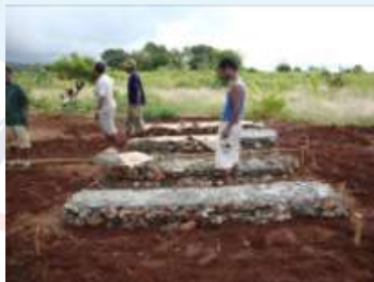
Building the foundation for the containers to sit on
