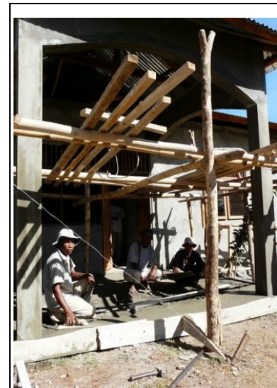
Our additional clinic building is nearing completion
